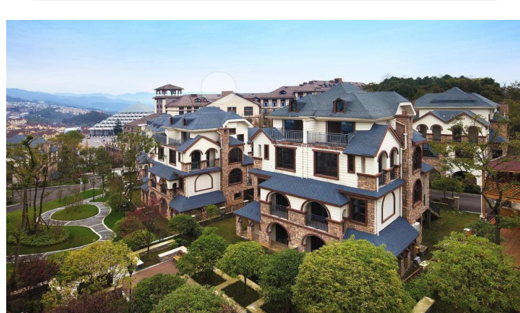
Villa area emergency power
